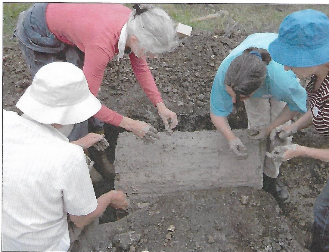
Plate 21: Roman kiln, building the flue arch
